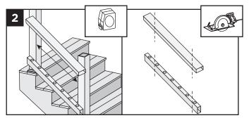
2. Set railing along the nose of the stair treads, making sure baluster holes are vertically aligned and mark line at each intersection. When measuring, cut equal lengths from each side of railing allowing a minimum of 2" on each end from the last baluster hole to the end of the rail. This will ensure proper baluster and bracket placement and equal spacing of balusters per each railing section.
