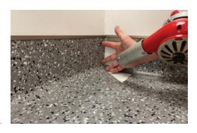
Warm your corner piece until it slides into place. Tape to secure and hold the warm corner piece in position until cooled.
