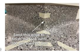
After the detail work is completed, use your adhesive and masking tape to hold the pieces in place until the adhesive has set. A small hand trowel or paint brush can work. Be careful not to over glue along seams.
