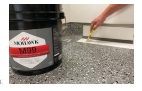
Continue to form the tile to complete your run of straight pieces. Let them cool, then apply the correct adhesive to all areas where the flash cove tile is positioned. Continue to tape the pieces together to hold tight seam.
