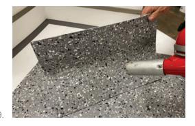
With your heat gun, warm the tile where the cove stick and the tile will meet until it becomes flexible. Keep the heat moving across the piece.
