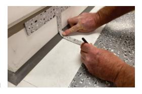
Repeat the same process as above on straight runs by marking the Tile - T against the installed tile floor. Tight to the radius. This will influence the high edges during cooling.
