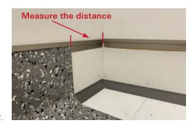
Measure the distance from the installed flash coved tile to the inside corner.
