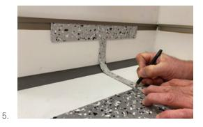
Using your Tile - T, push the flat edge under the cove cap following the radius until you meet the tile edge.
