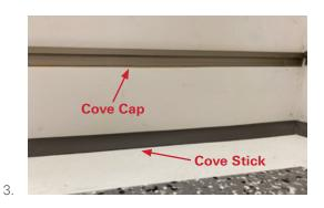
Install Cove Cap and Cove Stick, by using contact adhesive and 1 1/2" masking tape, staples or brads will work to secure. Let the cove cap and cove stick dry over night.
