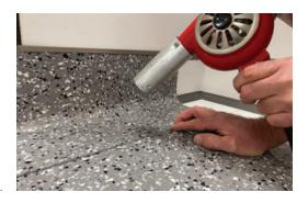
Continue to warm the tile until you have the tile in place. Using 1 1/2" masking tape, tape the tile to the installed floor edge as it cools to maintain the shape.
