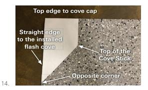
Cut out the piece and warm up the piece with a heat gun and install the piece. Adjustments are not uncommon.
