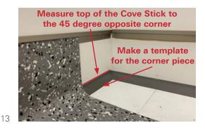
Make the first piece for the corner using a piece of paper to follow the contour of the wall.
