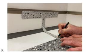
Using your pencil or marking device, put a mark on the Tile - T. This gives you the total height of the tile that will be formed.
