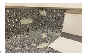
Warm up the corner piece, bending and adjusting the fit until the tile is in place properly. Tape the seams until the tile is cooled.
