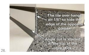
Dry fitting the outside corner pieces and modifications several times is needed for a proper fit.
