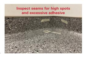
Hand roll and inspect any areas for seam movement. Clean and repair adhesive spills or seam blowouts. Follow clean up instructions on the adhesive label.
